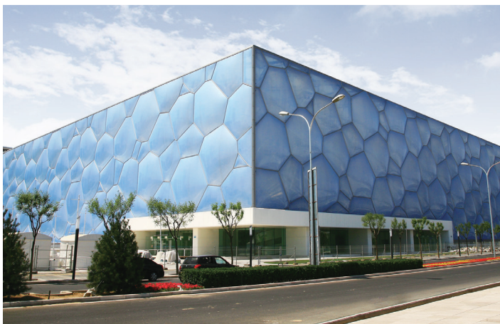
▲ Beijing Water Cube
